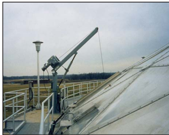
Left: Secondary tie off support secures the mixer in place. the davit raises or lowers the mixer into position.
