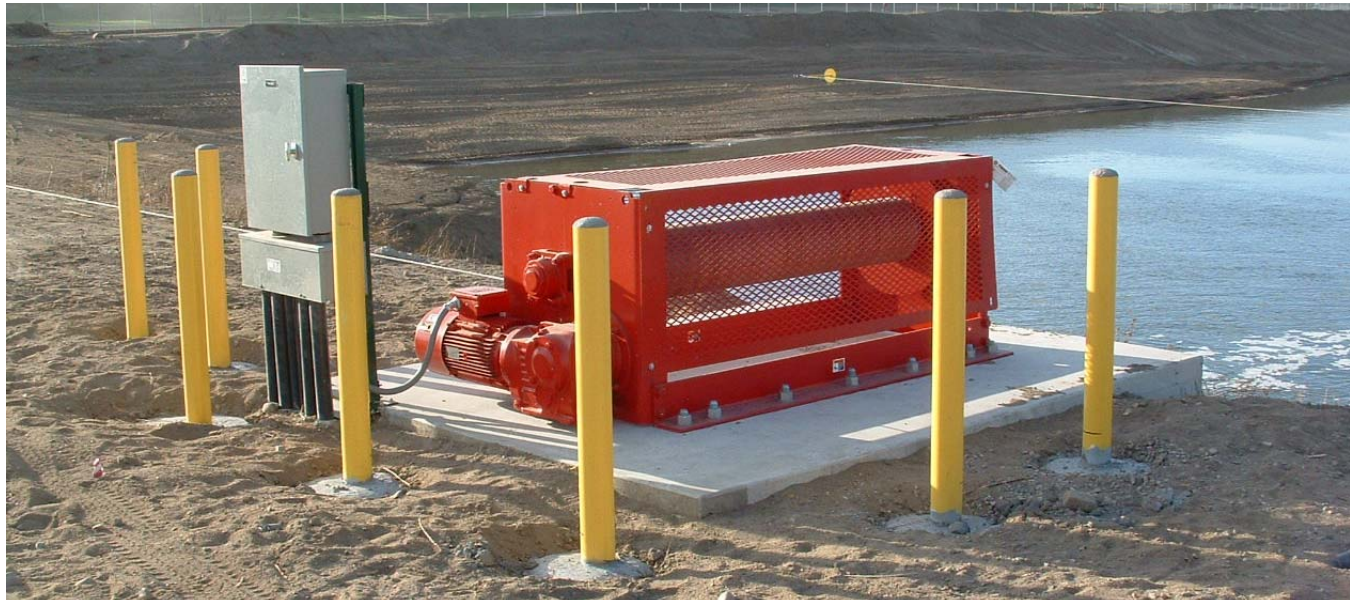
Above: The Orange County Water District built winch stations at each lagoon replacing older steel track systems. Winches connect to floating dredge units and maneuver them across the water, effectively removing silt deposits.
